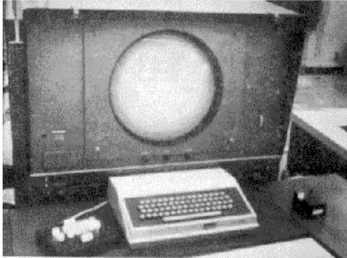
Figure 4. *Human-Machine Interaction at SRI with Keyboard, Push-Buttons, and Mouse, 1960s.*
